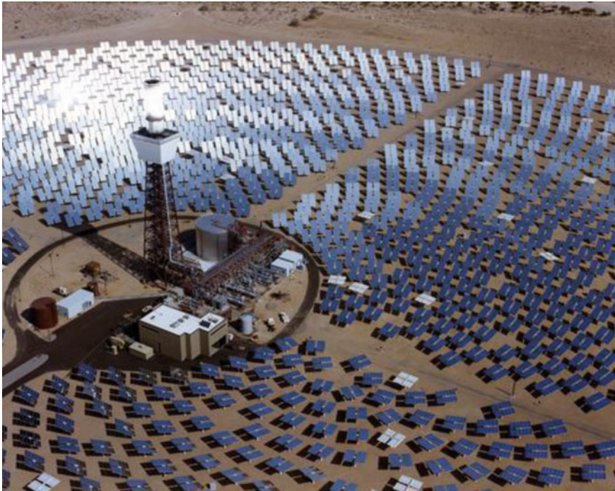
Fig. 7.7 An aerial photograph of Solar-Two, a 10 MW solar thermal plant near Barstow California (courtesy of Sandia National Laboratories)
