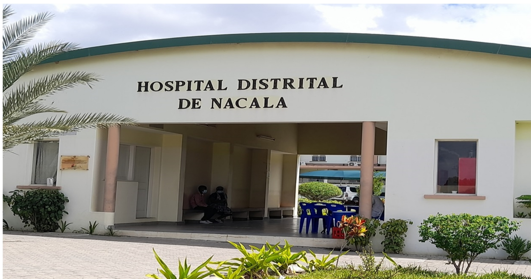
Figure 28: Hospital distrital de Nacala
